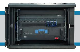
Telecor's wall cabinets provide ideal enclosures for eSeries equipment located in remote wiring closets.
